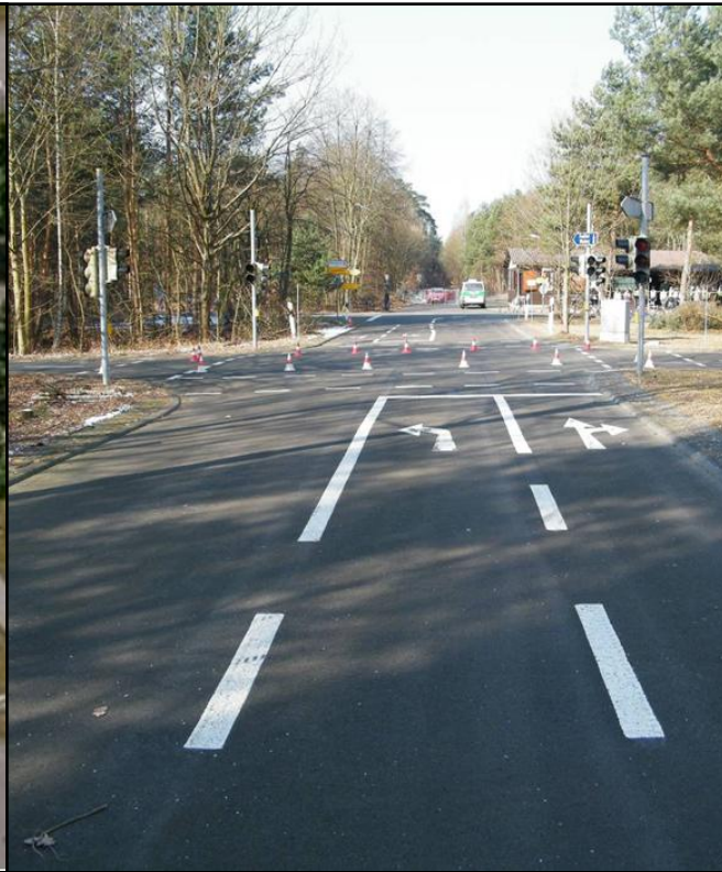
Test Intersection Alzenau
