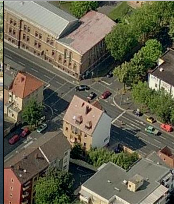
Public Intersection Aschaffenburg
